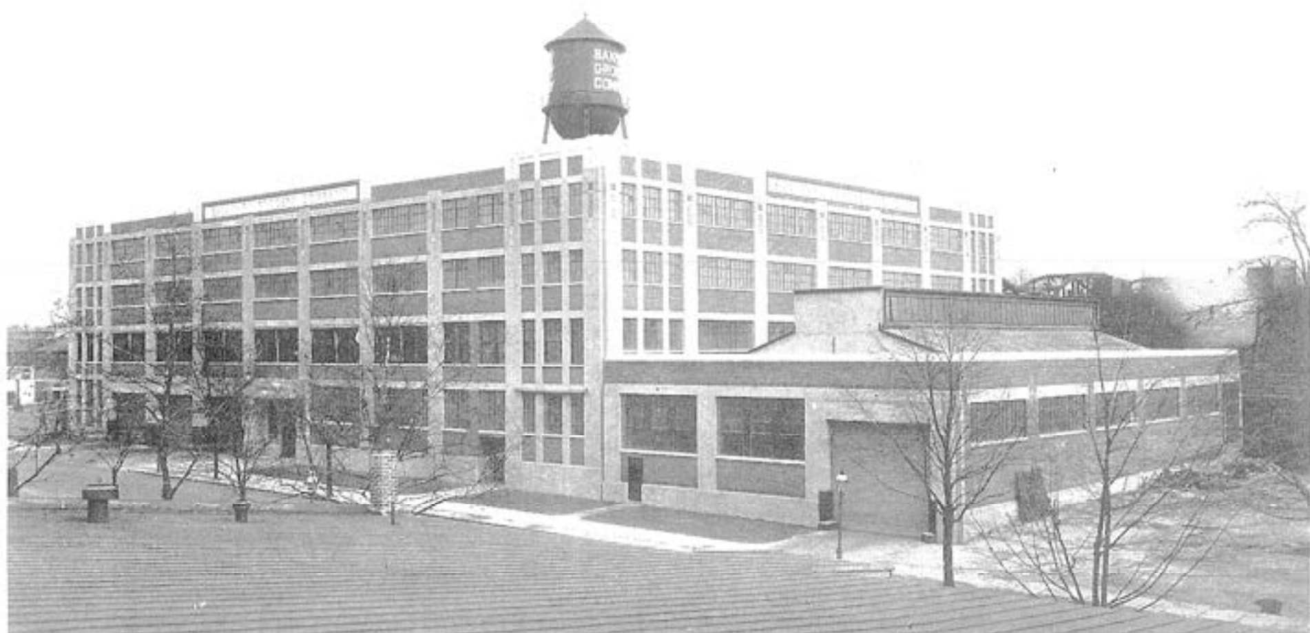
OFFICE AND WAREHOUSE, SAFEWAY STORES, INC., WASHINGTON, D. C.
