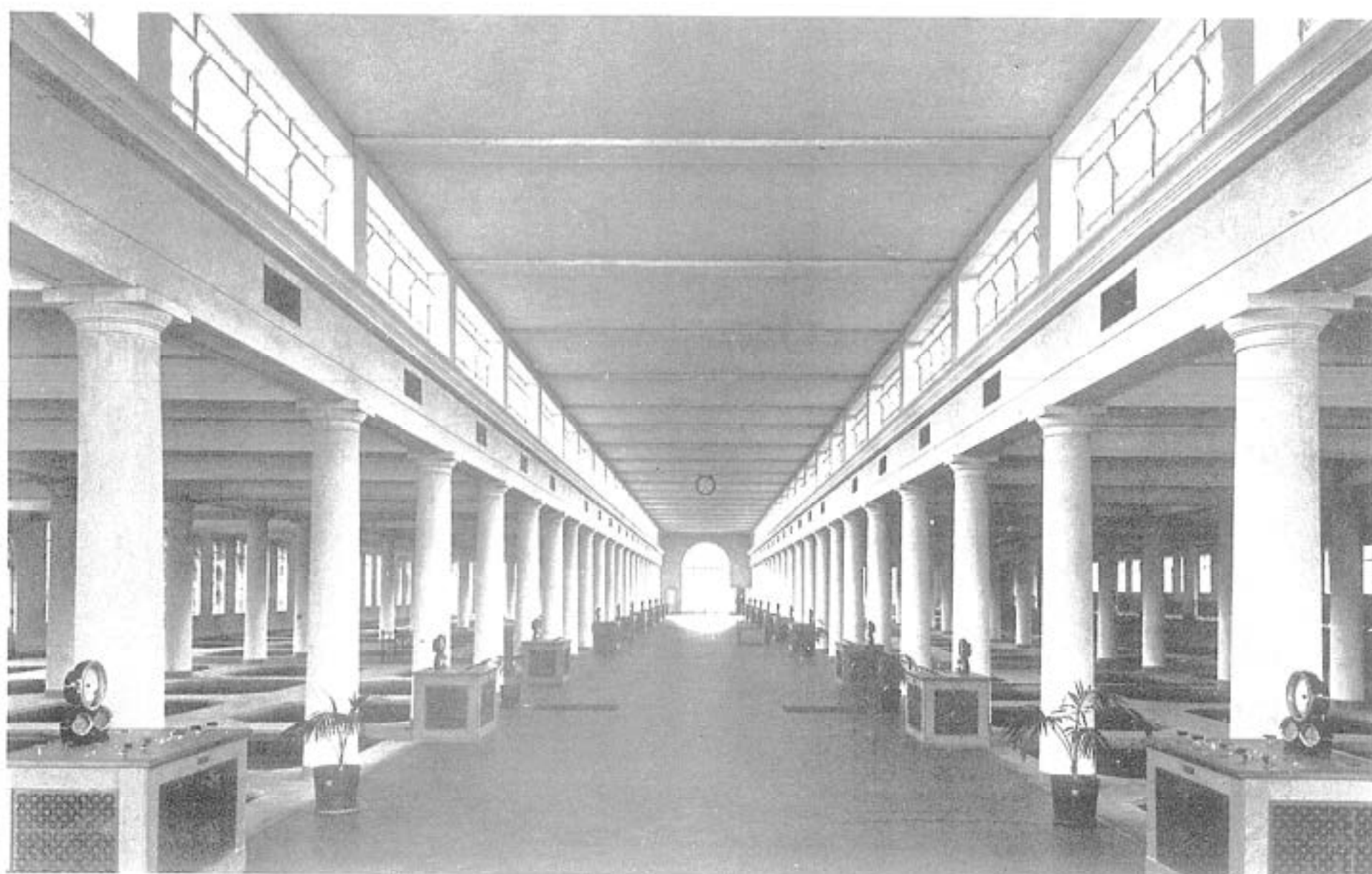
OPERATING GALLERY DALECARLIA FILTER PLANT, WASHINGTON, D. C.
