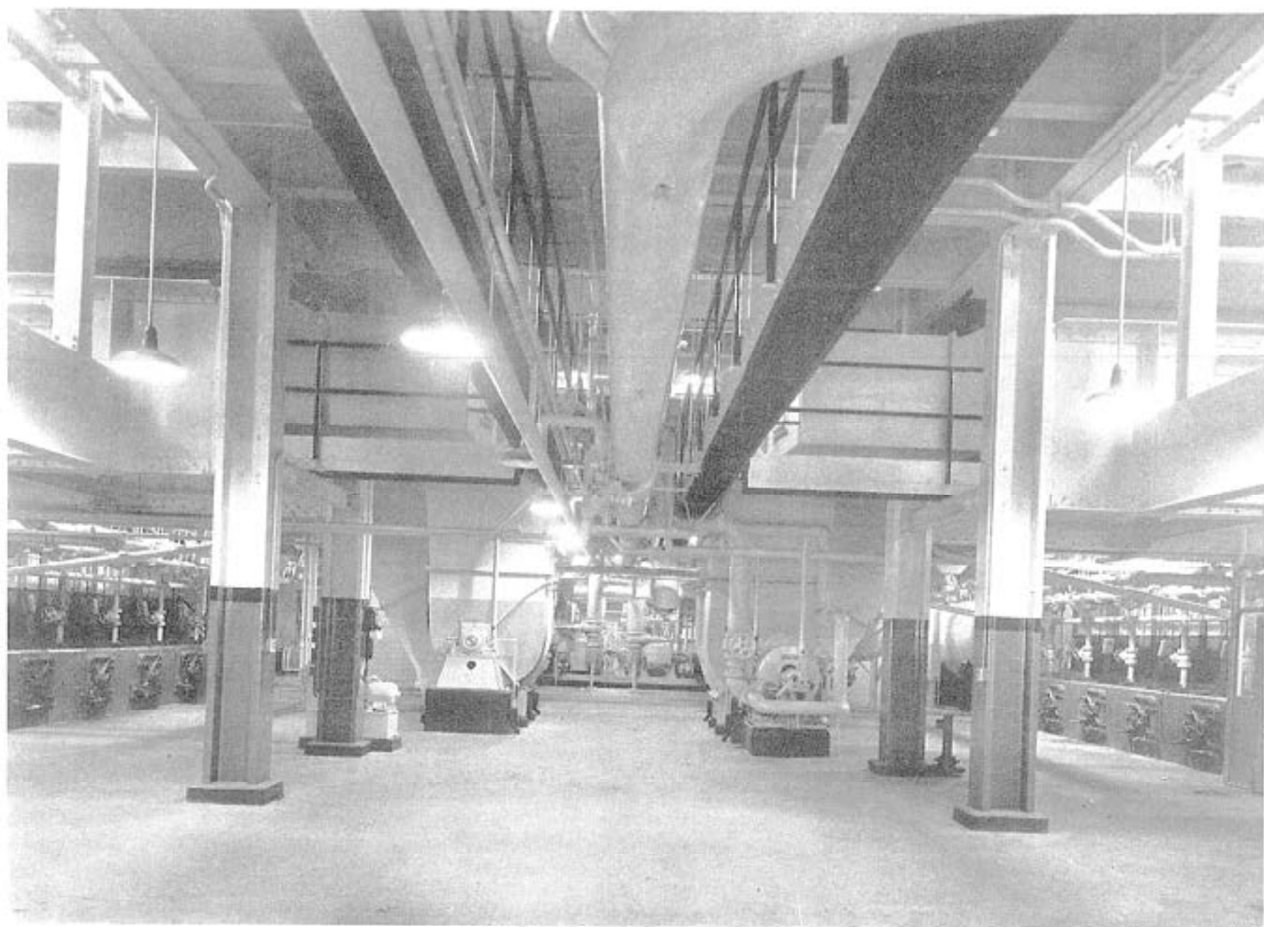
GROUND FLOOR, LOOKING WEST
