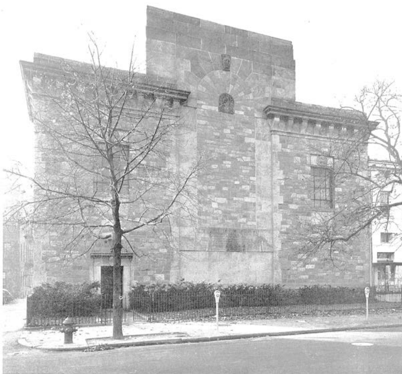
SUBSTATION, POTOMAC ELECTRIC POWER CO., WASHINGTON, D. C.
